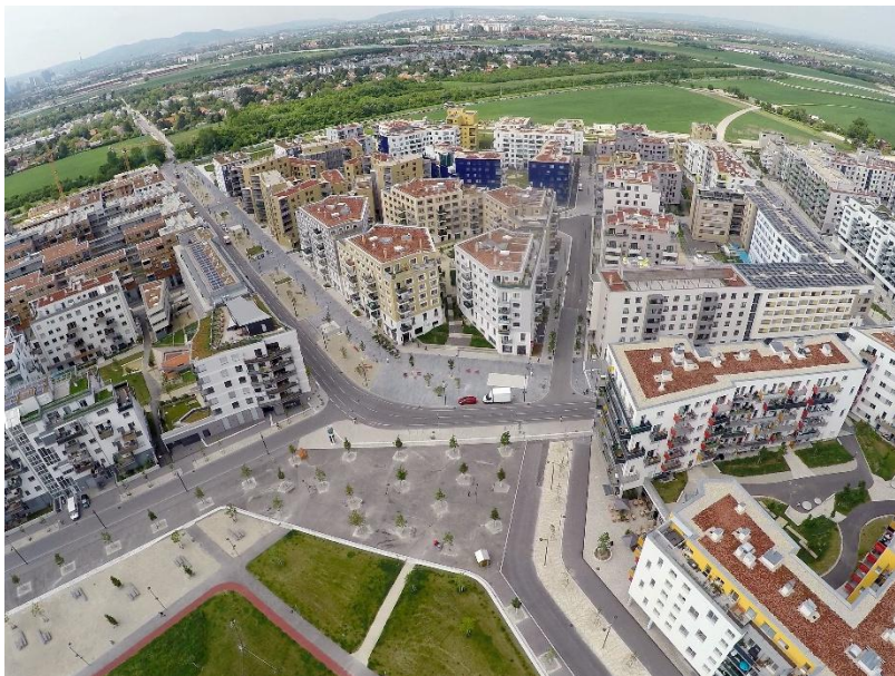
Aerial view Seestadt © ASCR, Photo: Walter Schaub-Walzer
