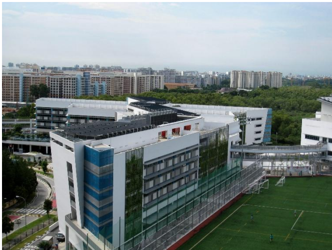
Solar heating and cooling of the UNITED WORLD COLLEGE, Singapore Photo ©: SOLID
