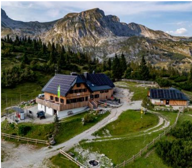
Drone shot of the Sonnenschienhütte, Photo: Imre Antal
